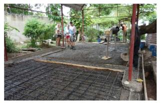
Constructing the blinding concrete. In the front: Finished reinforcement. Photo: Mareike Thiedeitz
